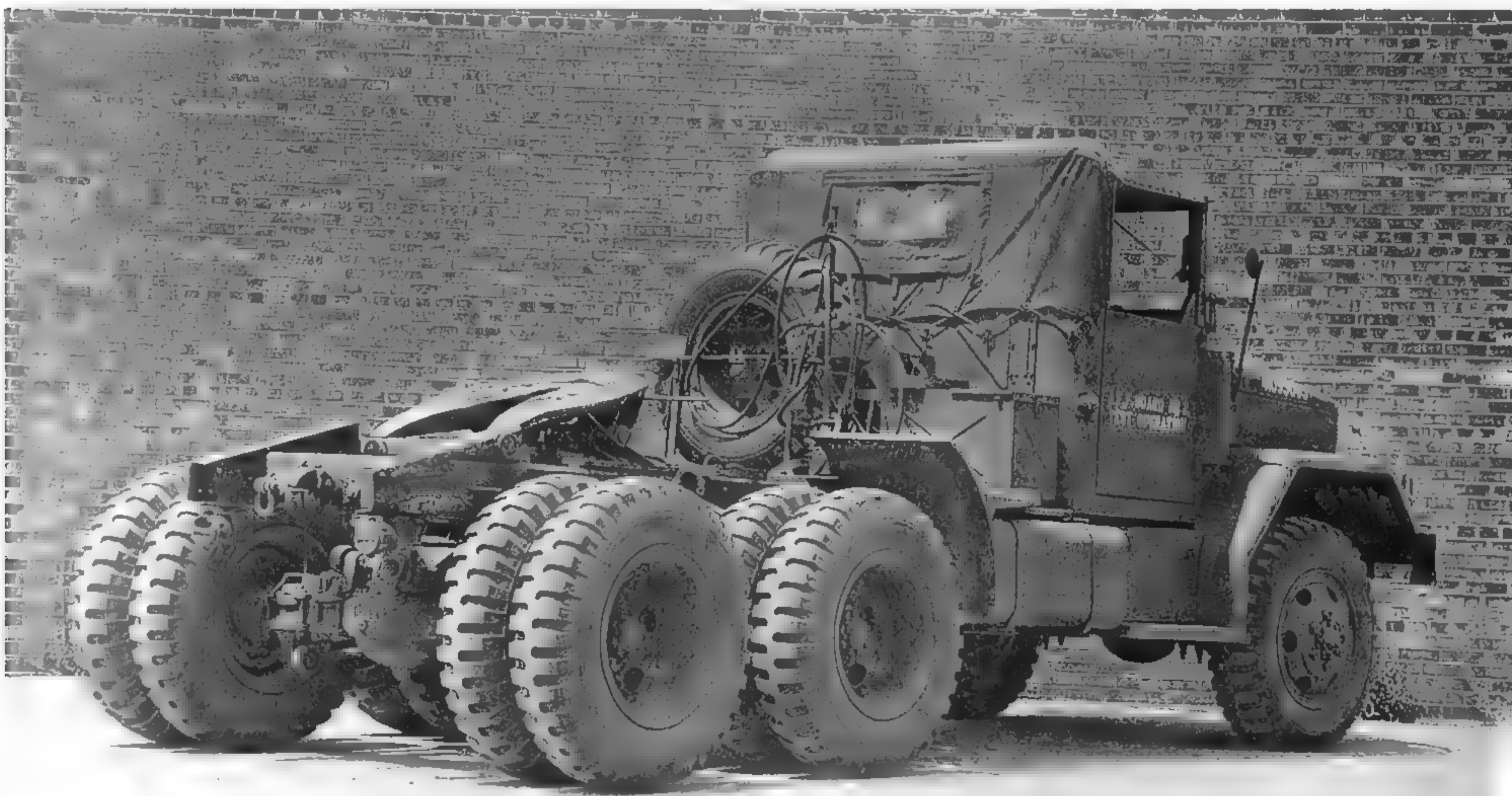
The fuel tank of the M275 series was a special long unit located on the driver's side in the space normally occupied by a M35's toolbox and spare tire. (Photo courtesy of John Winslow and Bruce Kubu)
